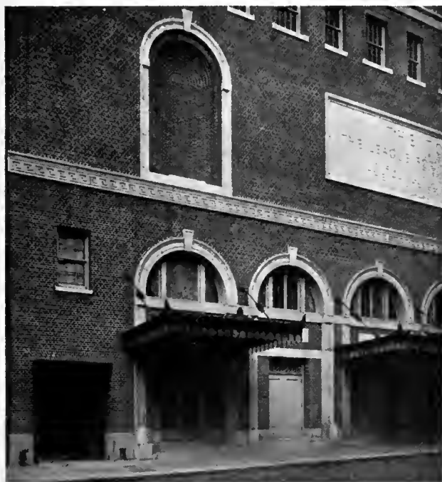
ENTRANCE DETAIL THE TOWN HALL, NEW YORK CITY McKIM, MEAD & WHITE, ARCHITECTS
